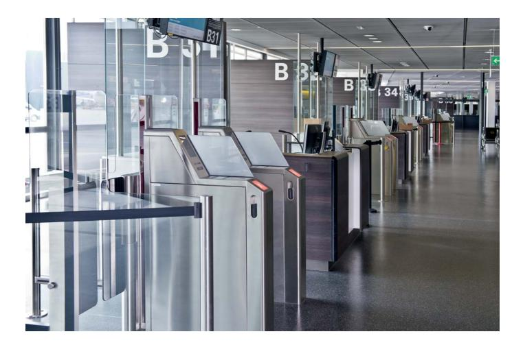
Waist-high sensor barrier, designed as an e-gate for self-boarding. Helps airport and ground staff keep the boarding process smooth and steady.
